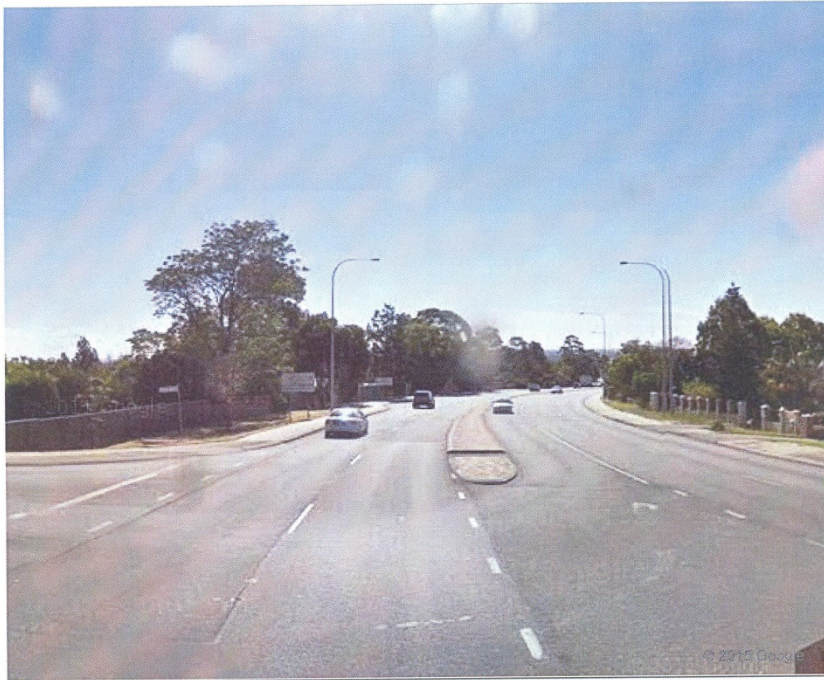
GRT EASTERN HWY AND SCOTT ST INTERSECTION, LOOKING NW
